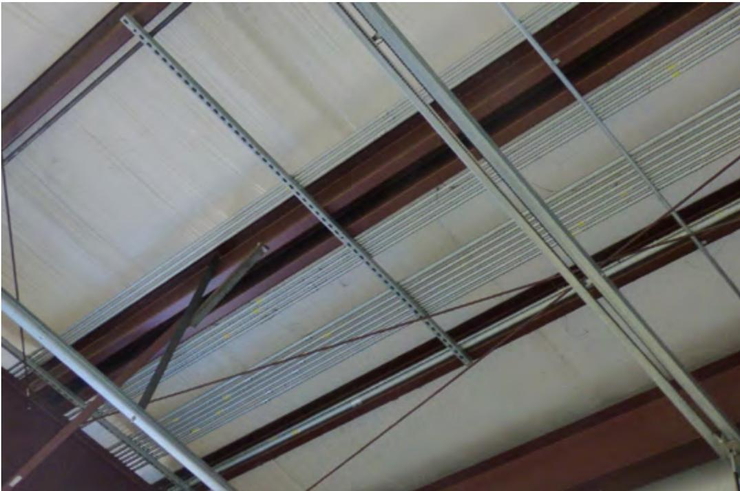
*Conduit within 18 inches of the ceiling is acceptable if it is sealed against gas migration. If it is unsealed, it could be a path of migration and may need to be relocated.*
