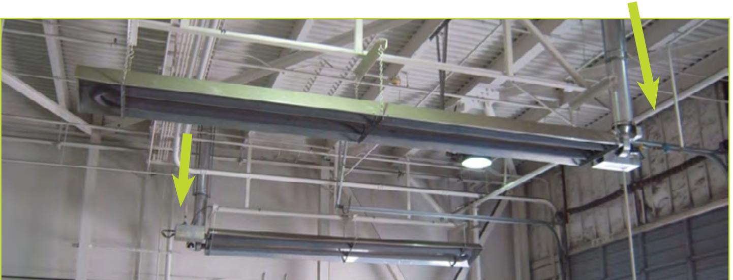
Compliance with the codes and regulations can be achieved by simply removing the non-compliant heating units and/or replacing them with units that are compliant. Gas-fired infrared tube-type radiant heaters are commonly employed in maintenance facilities that service conventionally fueled vehicles. Manufacturers of these types of heating systems now manufacture units that have contained flames and surface elements that do not exceed 750°F and sealed combustion chambers.
