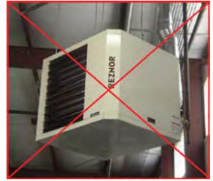
**Localized space heating is another method for heating a maintenance facility. Localized space heating is typically accomplished using open flame gas-fired, infrared, direct radiation, tube-type heaters fueled by natural gas or propane, or electric infrared heating units. Most of these types of heating apparatus are mounted to either the wall or roof of the facility or suspended from the ceiling.**
